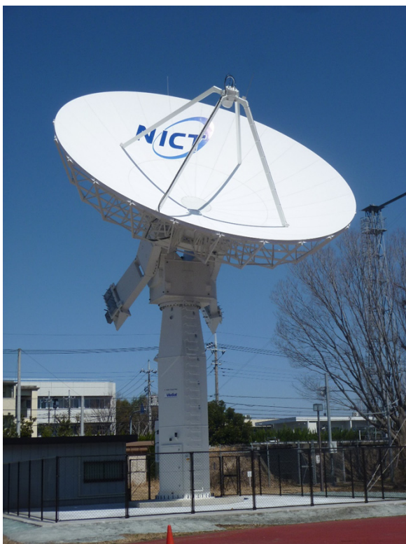
The 11.3 meter antenna system to receive real-time solar wind data from ACE and DSCOVR
