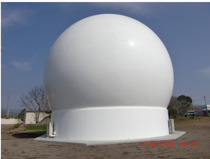
The 16 meters in diameter radome. The radome shields a parabolic antenna from typhoon and volcanic ash
