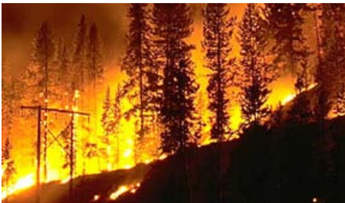
Figure 4. Wildfire disrupting electricity transmission
