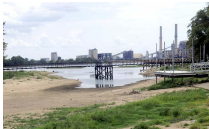
Figure 11. Low water level at Martin Lake Steam Electric Station facility in Texas
