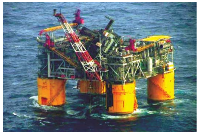
Figure 20. Damaged offshore platform after Hurricane Katrina
