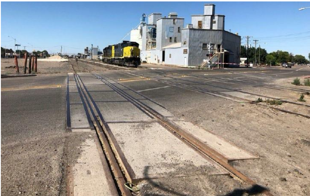
SH-24/8 th Street in Rupert, ID. EIRR Magic Valley Rail Safety and Capacity Expansion.
