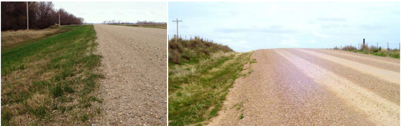
Figure 11: Examples of good gravel shoulders.
