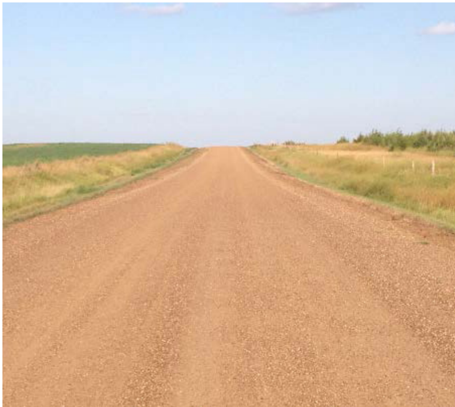
Figure 8: Gravel road with adequate crown.
