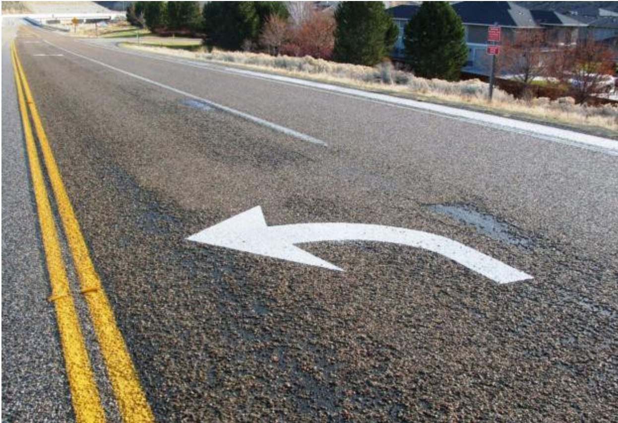
Design: Chip Sealing on newly paved asphalt pavement; unacceptable chip loss (CODs)
