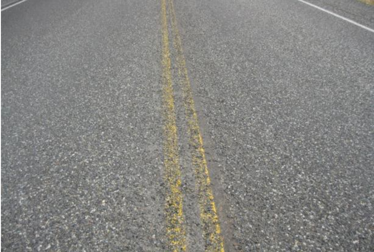
Longitudinal Joint: Acceptable chip loss
