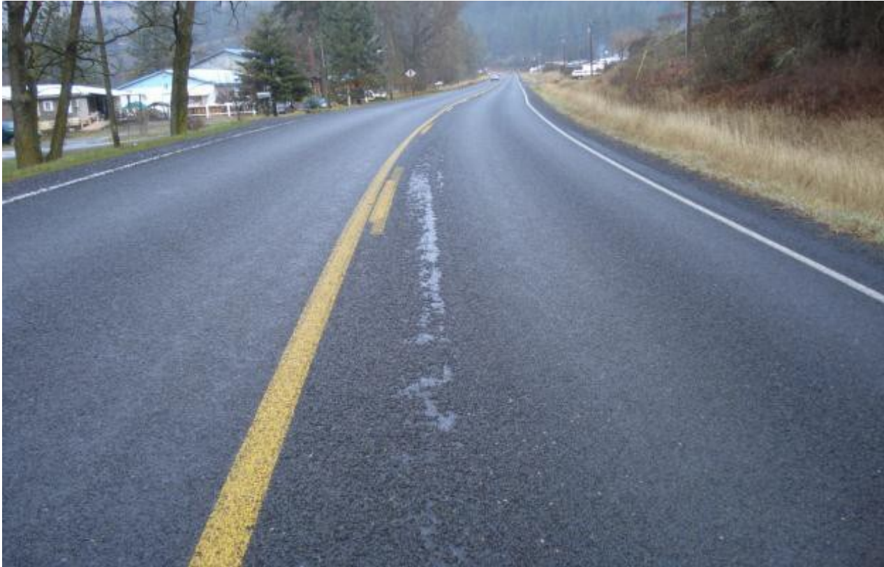
Plugged nozzle: Acceptable chip loss
