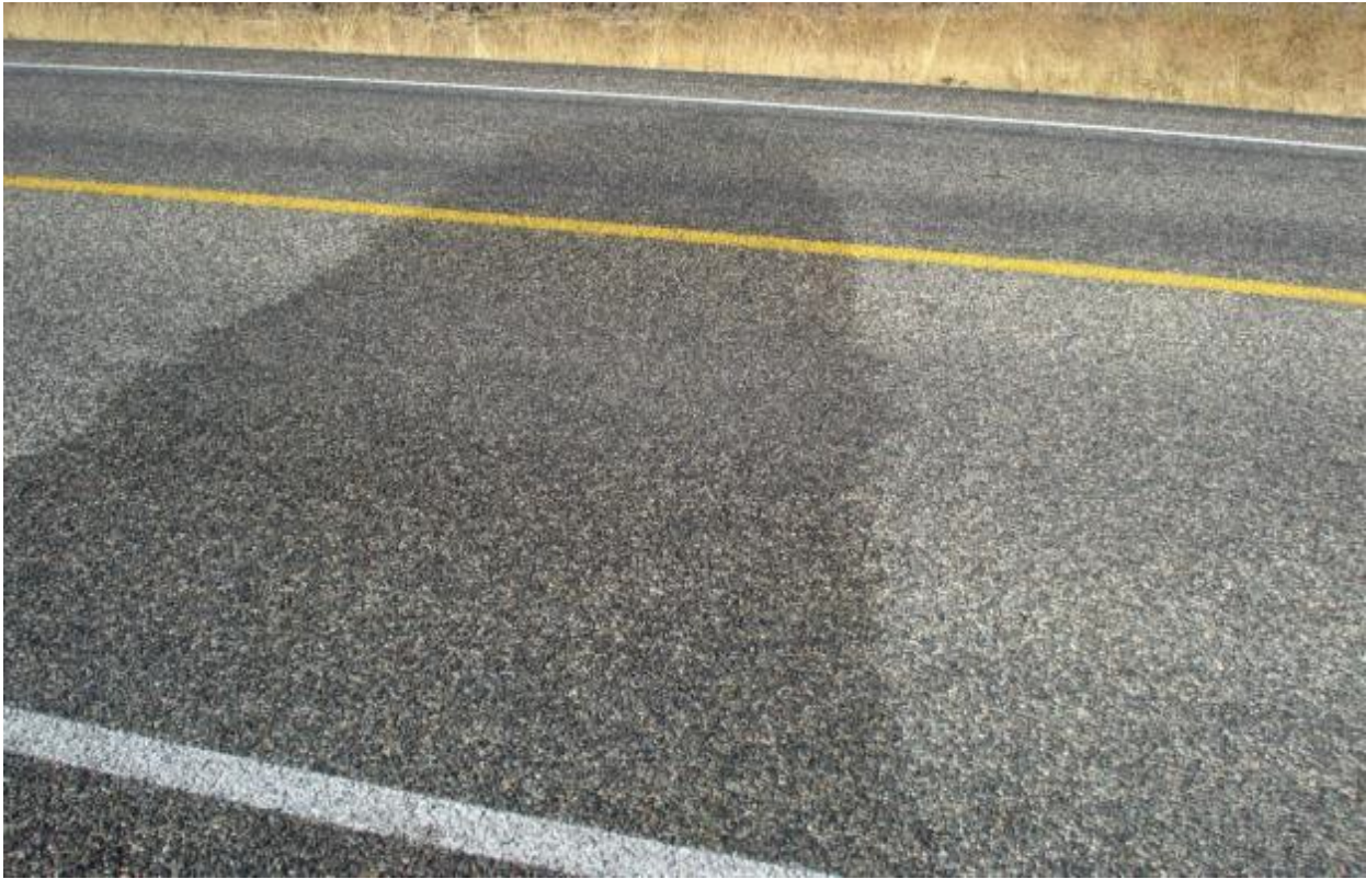
Traffic: Tire chain damage (NCODs)
