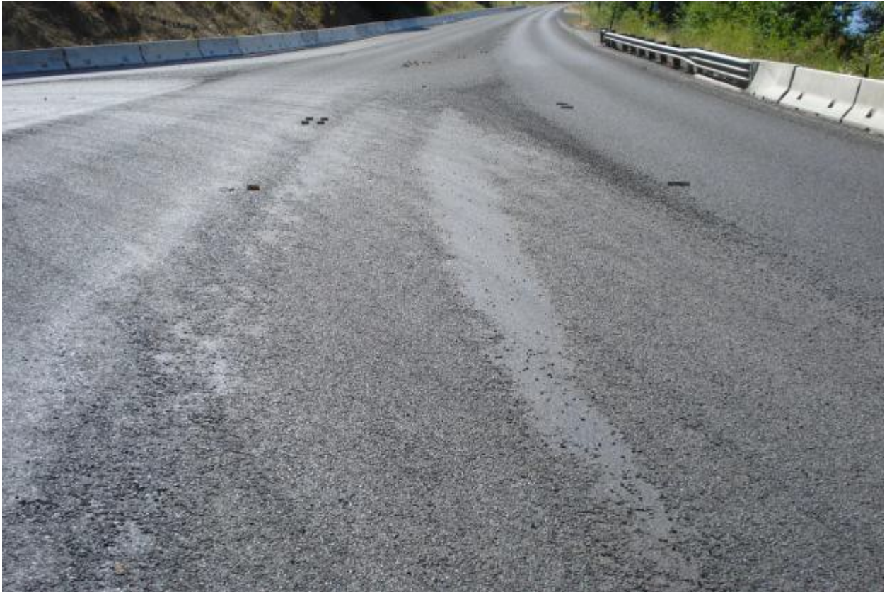
Traffic: Chip loss from turning movements (CODs)
