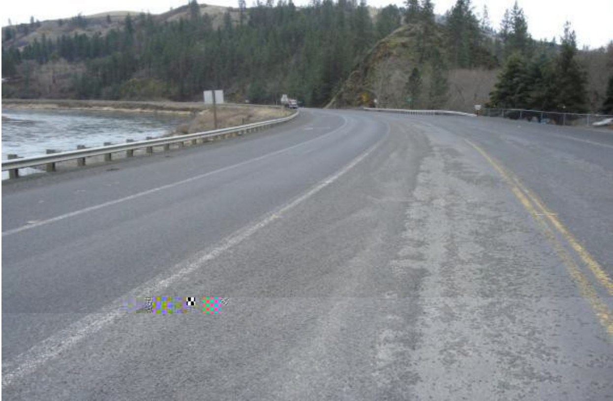
Design: Chip Sealing on newly paved asphalt pavement; unacceptable chip loss (CODs)
