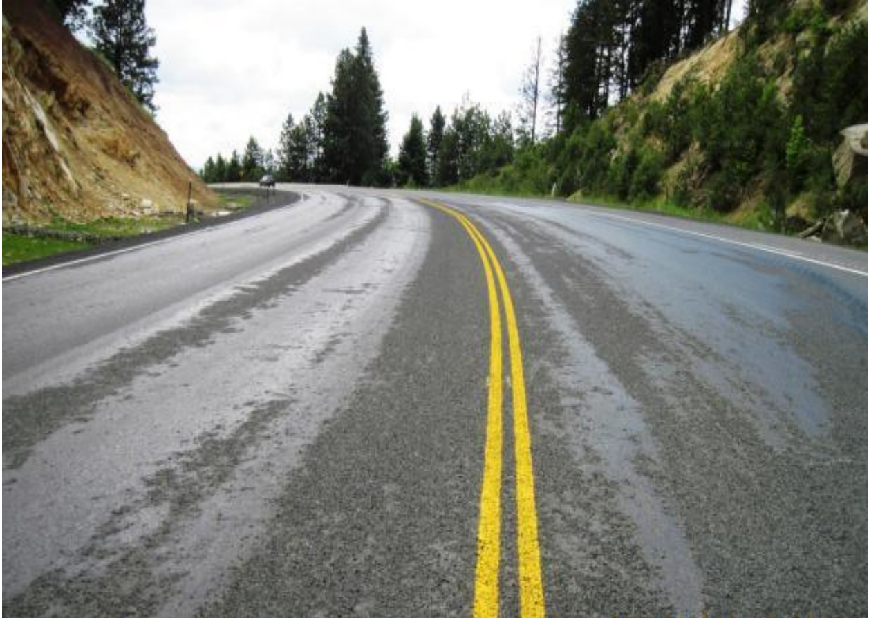
Weather: Rain and cool weather following construction, unacceptable chip loss (CODs)
