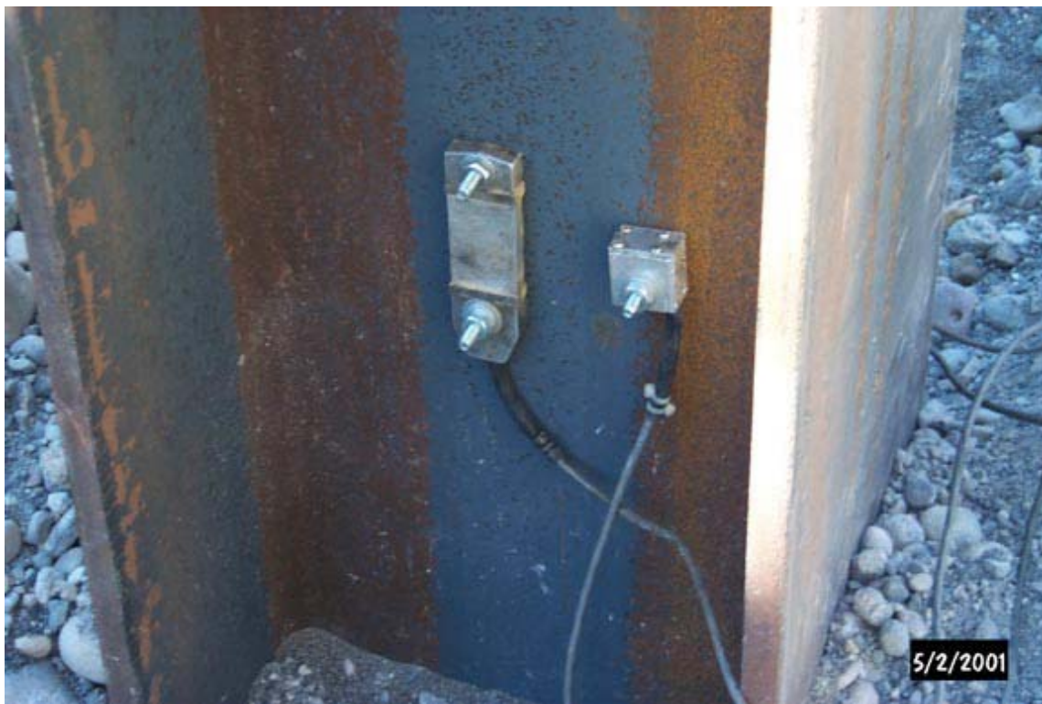
Photo 5. PDA transducers attached to pile.
