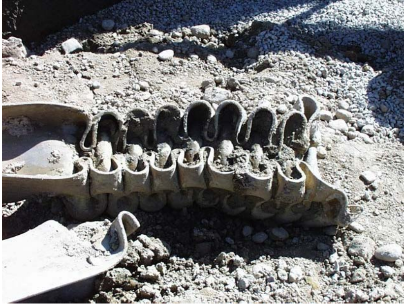
Photo 3. Damaged H pile due to overdriving.
