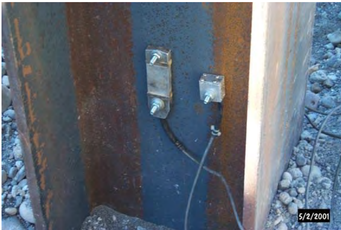
Photo 5. PDA transducers attached to pile.
