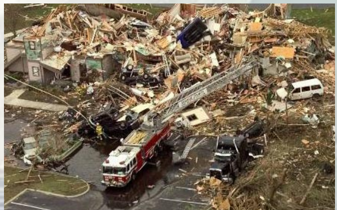
Tornado damage, Winter Garden, Florida, February 1998
