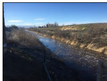
Figure 47 – Sulphur Creek Wasteway downstream view
