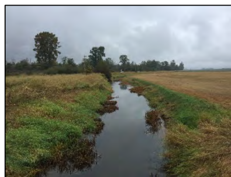
Figure 8 – Lower Big Ditch upstream view
