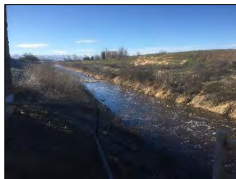
Figure 47 – Sulphur Creek Wasteway downstream view
