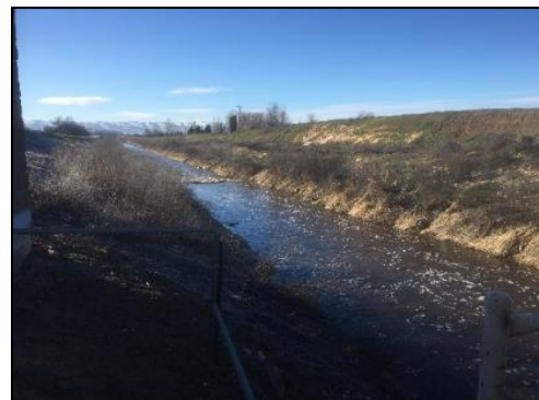
Figure 43 – Sulphur Creek Wasteway downstream view
