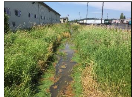
Figure 8 – Upper Big Ditch upstream view
