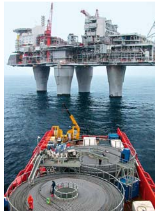
Troll-A oil platform in the North Sea and cable laying ship (ABB)
