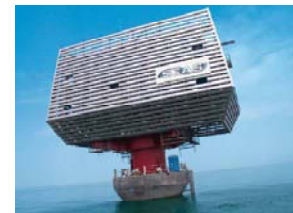
Transformer unit (33 kV/132 kV) for the aggregation of the 72 wind turbines of the park, 165 MW
