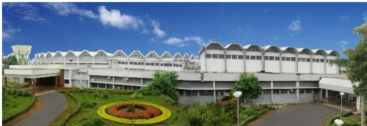
Indus-1 & Indus-2 Synchrotron radiation facility at RRCAT
