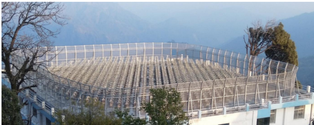
Figure 6: A bird-eye view of ARIES ST Radar on the roof-top of the building.
