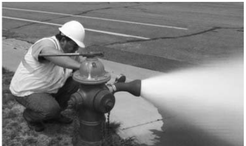
Figure 7.4.2. Flushing hydrants
