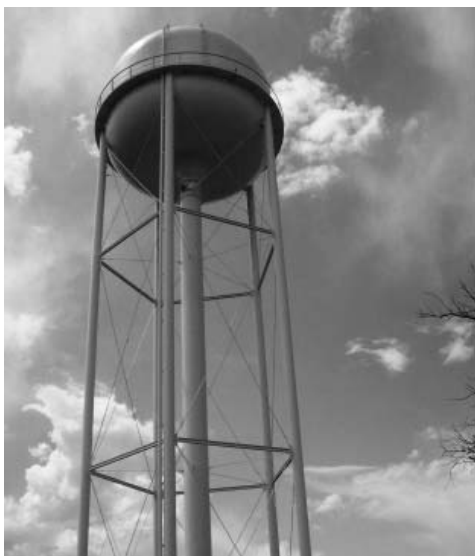
Figure 7.1.5a. Elevated Steel Tank
