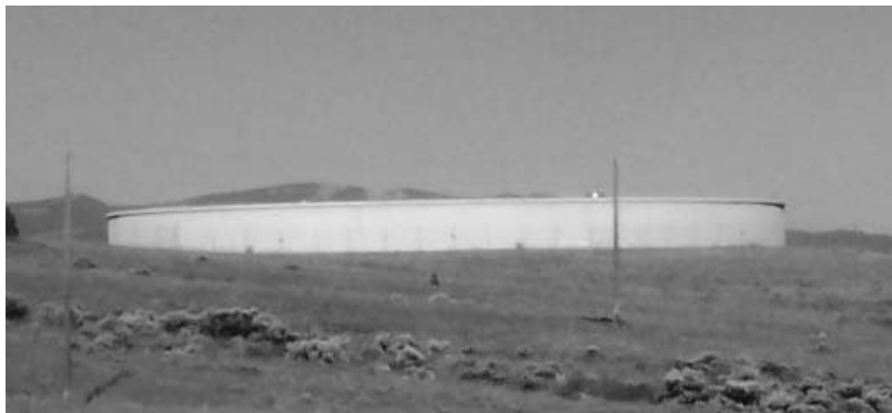
Figure 7.4.4. Ground-Level Storage Tank
