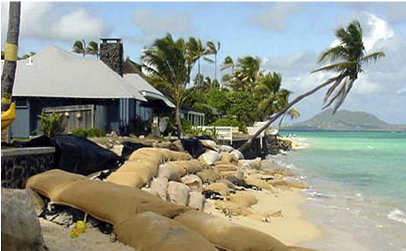
Figure 8. Insufficient shoreline setbacks often lead to armoring eroding shorelines - here shown with temporary geotextile bags.
