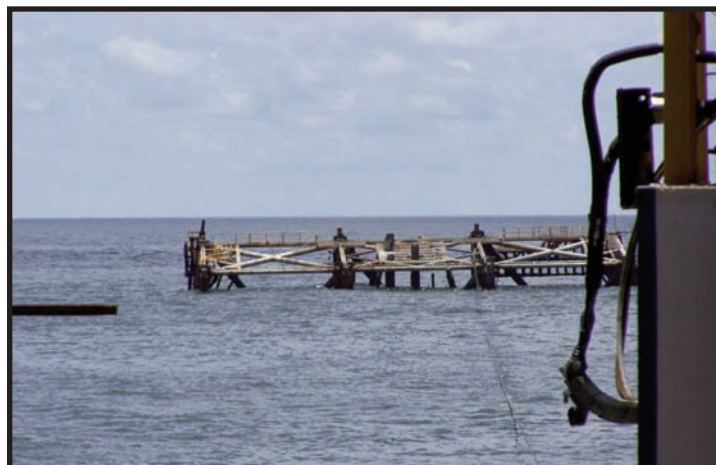
The Artificial Reef Bureau worked with Apache Corporation to deploy Main Pass 290 rig jacket for an offshore artificial reef.
