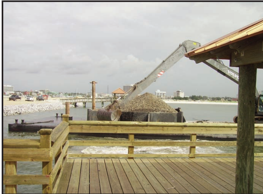
Emergency Disaster Recovery Program funds are being utilized to restore and diversify nearshore and offshore ecosystems through artificial reef habitats. Shown here is limestone being deployed near Urie Pier in Gulfport.
