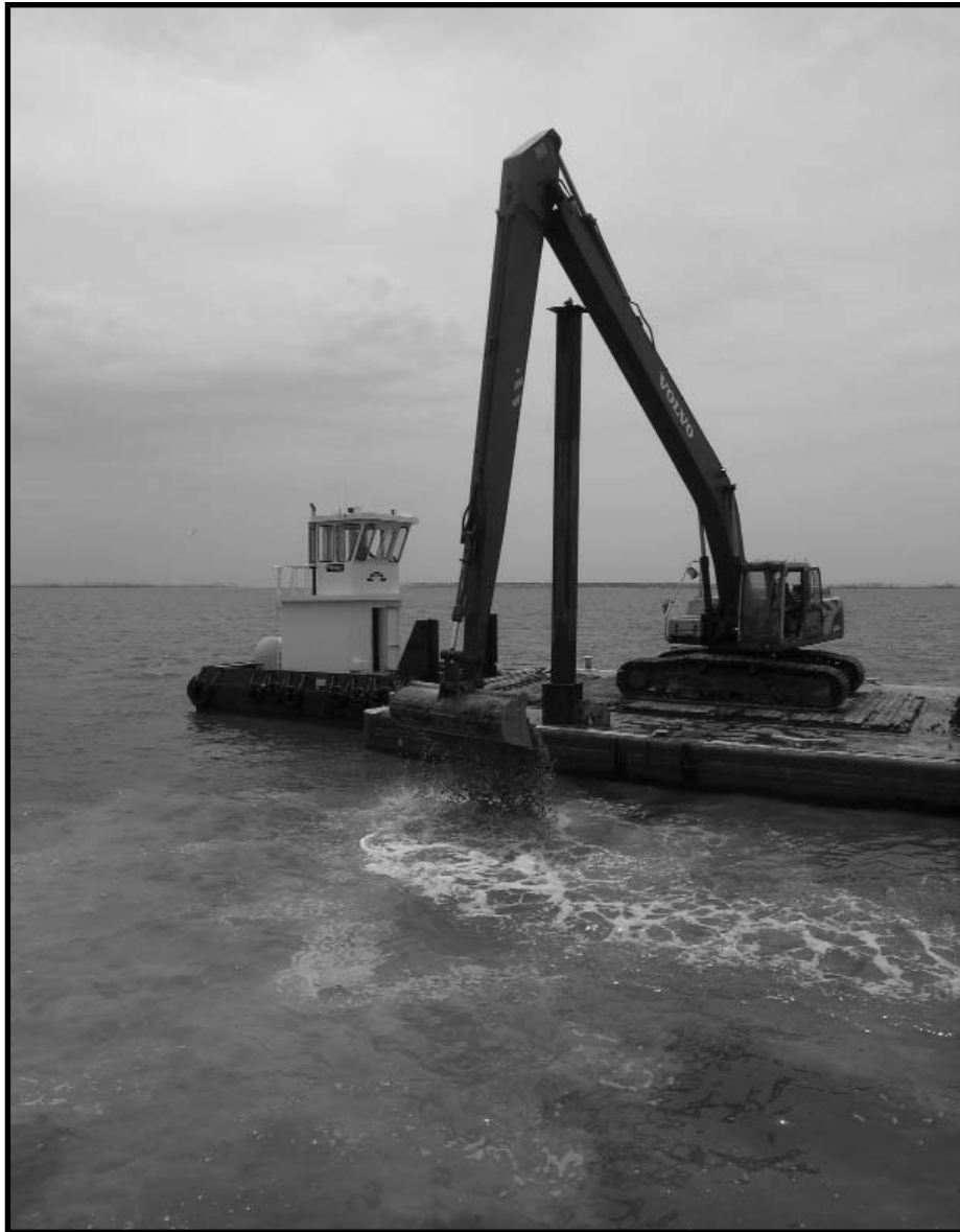
Crushed limestone is spread along the water just off the Ocean Springs Chester M. McPhearson Jr. community pier in July 2009 as part of the effort to restore artificial reef habitat destroyed by Hurricane Katrina. By early 2010, Mississippi's inshore artificial reefs had been restored to more than 100 percent.
