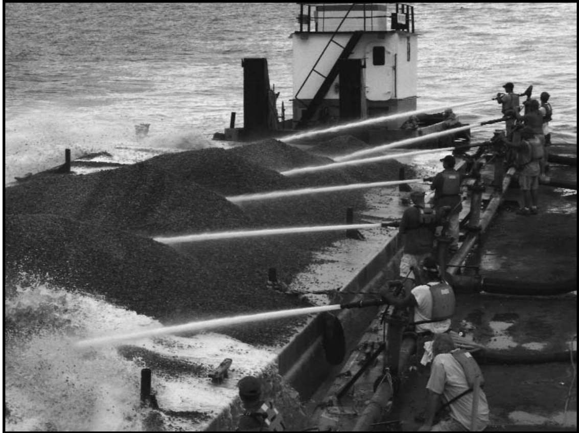
High-pressure hoses are used to spread oyster shells in August 2009 as part of the effort to rebuild Mississippi oyster reefs.
