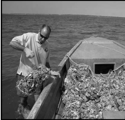
The Coastal Preserves Program and the DMR Shellfish Bureau worked together to create a berm/breakwater of oyster shell bound in metal mesh bags along the northern shore of Deer Island to protect the shoreline from erosion.
