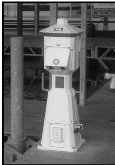
A standalone slip-to-slip pump-out unit provides boaters with a convenient method of pumping out.
