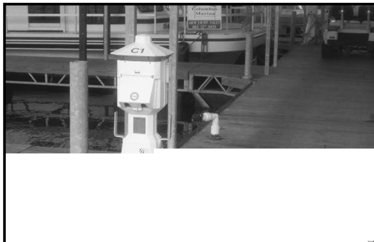
A standalone slip-to-slip pump-out unit provides boaters with a convenient method of pumping out.
