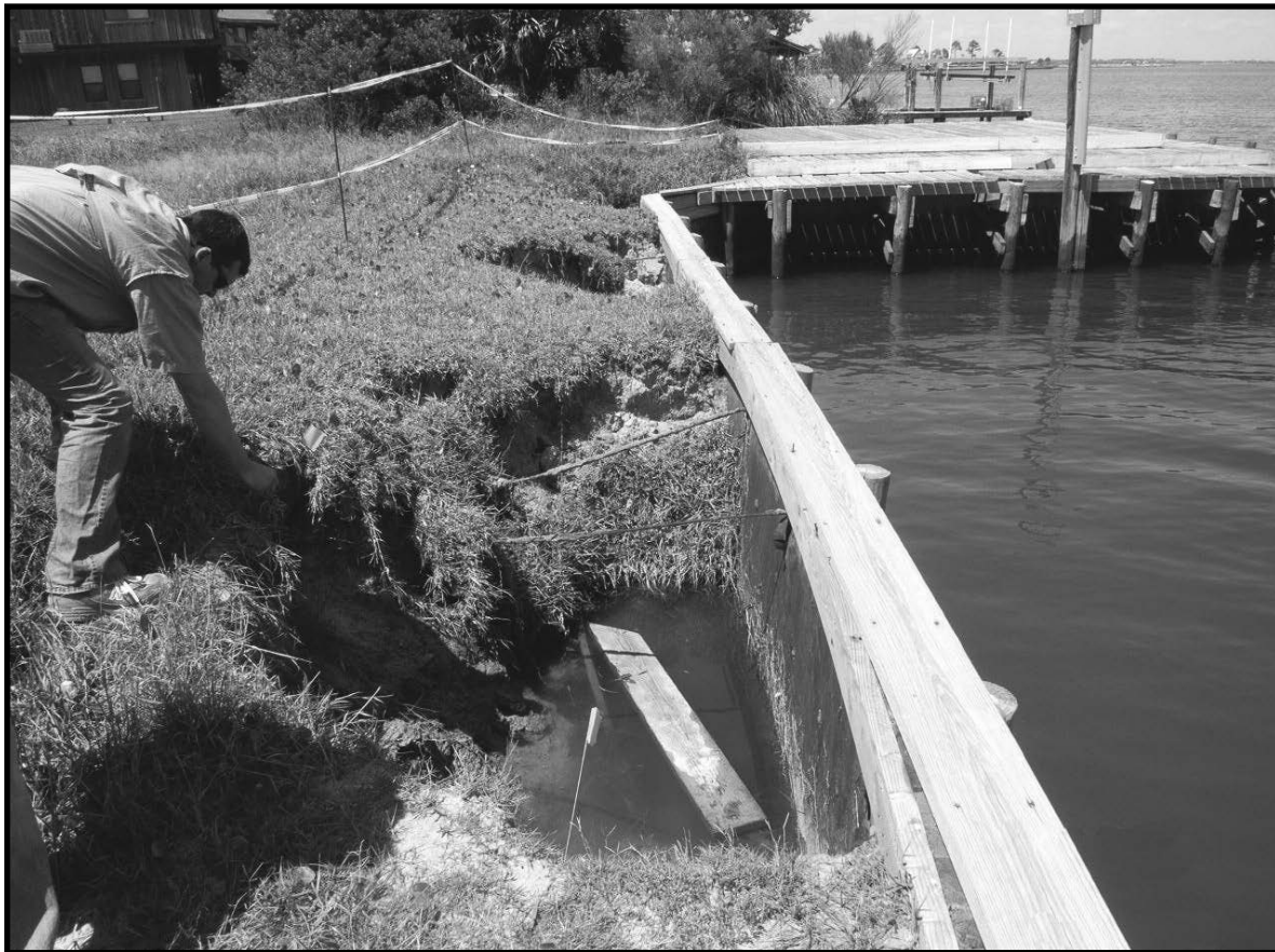
Jeremy Overstreet with MDMR's Permitting Program places flags for a bulkhead location.
