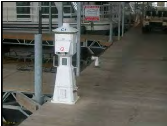
A standalone slip-to-slip pump-out unit provides boaters with a convenient method of pumping out.
