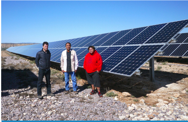
Regional Administrator Jared Blumenfeld, Tribal Council Member and Environmental Director Tommy Siyuja, Sr., and Augie Hanna visit a new solar array at the Havasupai Tribal School. This array will help save the Tribe money and energy, prevent frequent outages, and reduce greenhouse gas emissions. CREDIT: EPA
