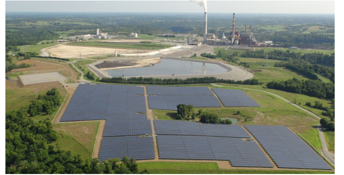
Figure 7. The LG&E and KU E.W. Brown universal solar facility, which houses a 14MW dc 10MW ac PV system. The PV system is divided into ten sections with each rated 1MW ac .
