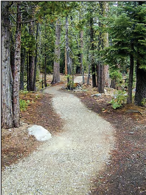
Trail Class 4: Constructed Features —Constructed features are frequent and substantial. Trailside amenities may be present.
