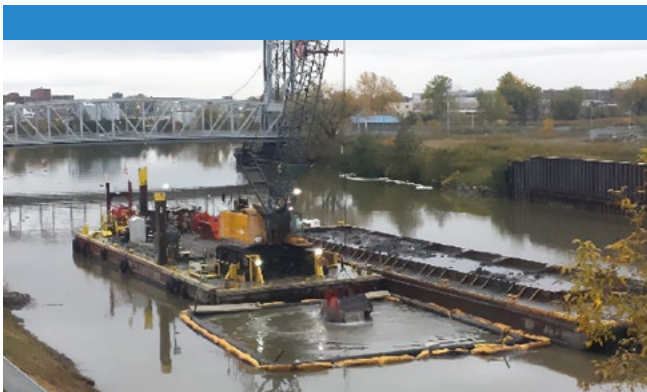
Mechanical dredging of contaminated sediment in the Buffalo River. Photo credit: Brian Murphy
