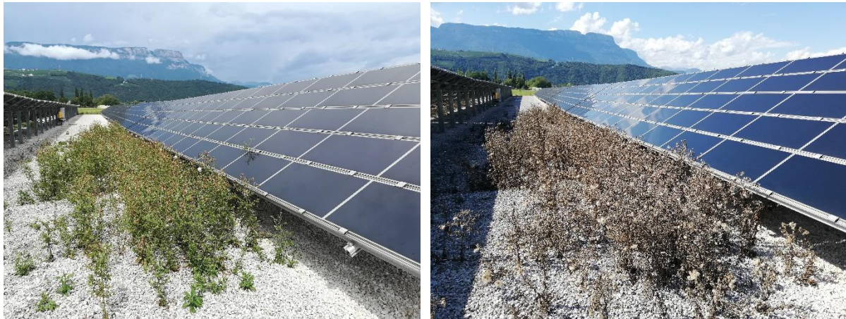
Figure 18: Vegetation before (left) and after spraying the herbicide (right) in a white stone ground [EURAC Research].
