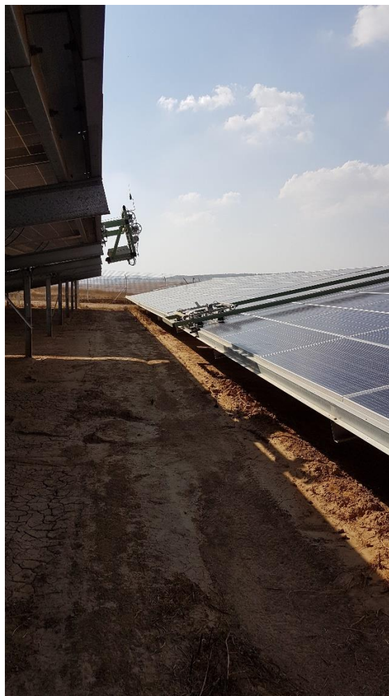
Figure 19: Automated cleaning of soiled PV modules in the Negev Desert, Israel.
