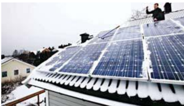
Figure 53: Brushing to remove snow from solar roofs [167].
