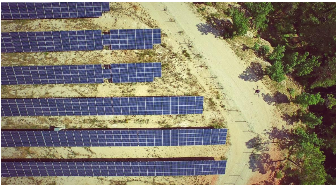
Figure 10: Aerial visual imagery for general inspection in general site management of a PV plant © CEA-INES.
