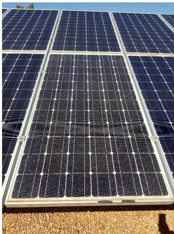
Figure 21: PV module damaged during vegetation management due to pebbles. Array in Central Australia.
