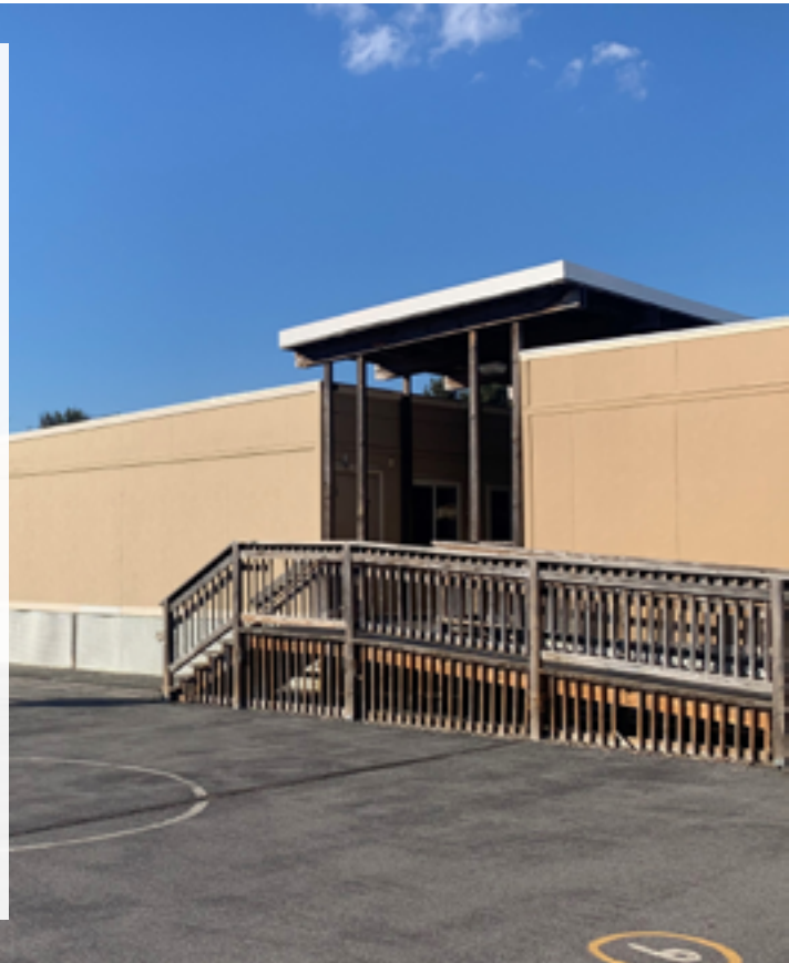
A TEMPORARY SCHOOL BUILDING IN MARYLAND.
