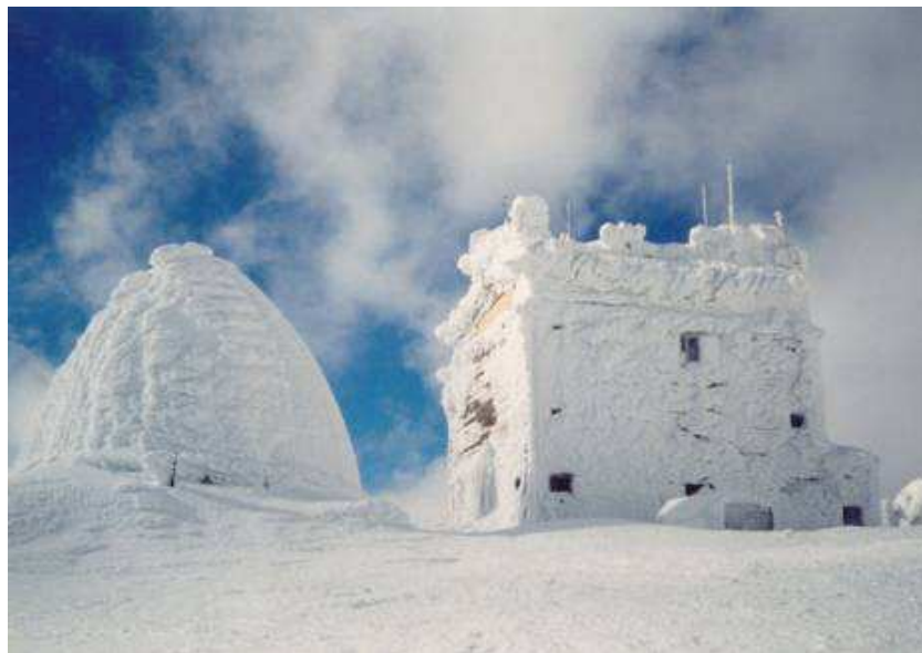
Fig. 4. Botev Peak station – a test site for the COST 727 Action project.
