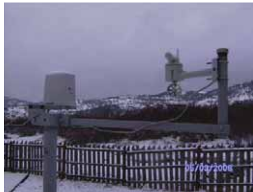
Figure 4. A part of the meteorological station installed at PLO4
