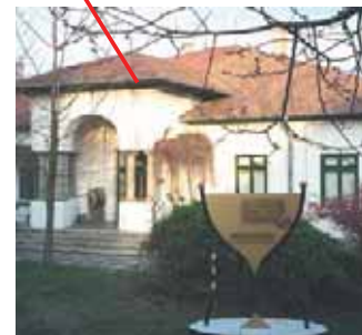
Caldarusani Geodynamic Observatory
