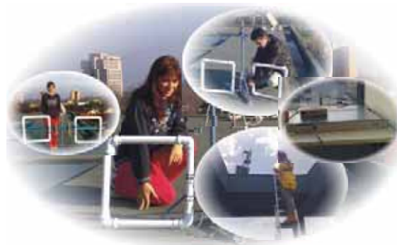
Figure 5. Magnetic VLF and LF antennas installed on the roof of the Dobrudja Observatory
