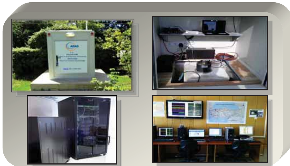
Figure 6. Main Server and Data Process Center.
