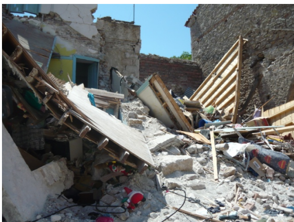
Collapsed buildings in Vrissa village (Lesvos Island, 2017)
