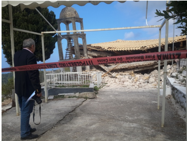
Damages in buildings and churches (Southern part of Lefkada Island, 2015)
