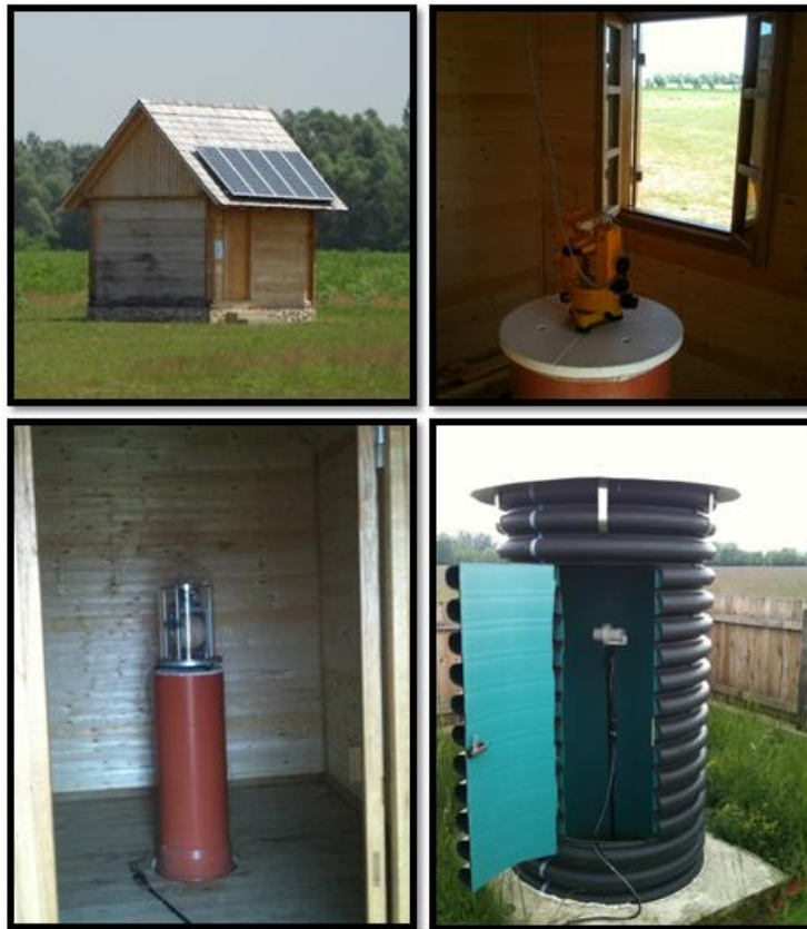
Figure 2. Top left: control house with solar cells on the roof; top right: geomagnetic theodolite; bottom left: dIdD magnetometer; bottom right: proton magnetometer.
