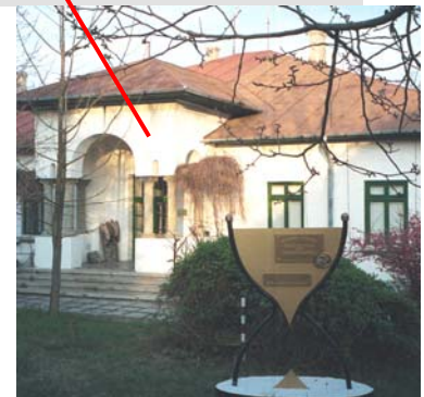
Caldarusani Geodynamic Observatory
