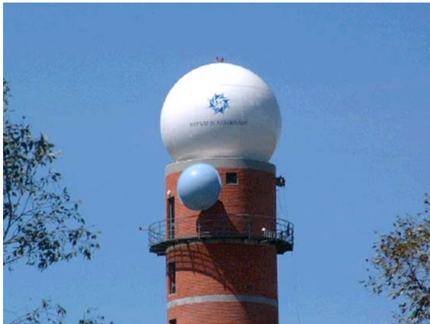
Cavalos do Caldeirão weather radar station (Faro), showing both the radar and radiolink radomes
