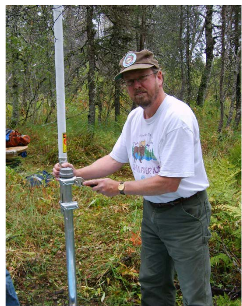
Installing equipment on an antenna mast, Dillingham, Alaska
