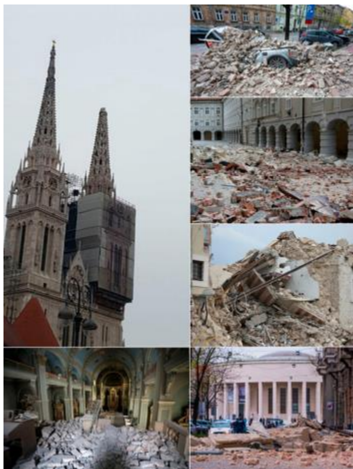
Figure 1. Photos of damage in Zagreb caused by the 22 March 2020 earthquake (from Markušić et al, 2020).
