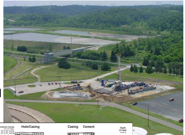
Drilling Test Well
