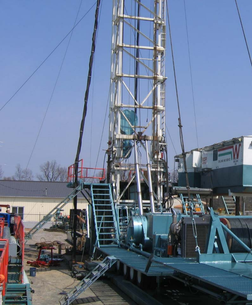
Rig for deep drill holes
