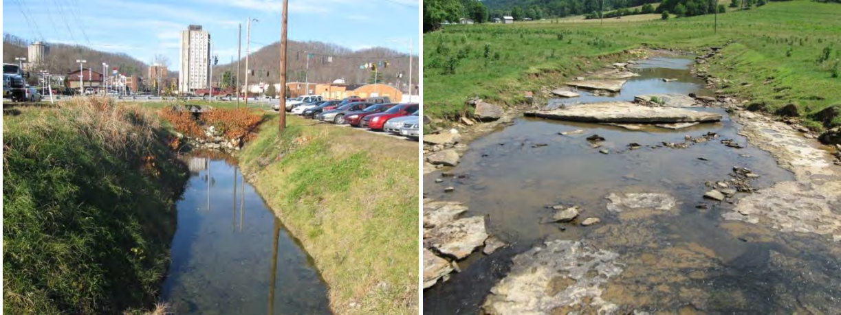
Figure 3.47. Photos of the two worst sites, EB-0.04 (left) and IF-0.05 (right).
