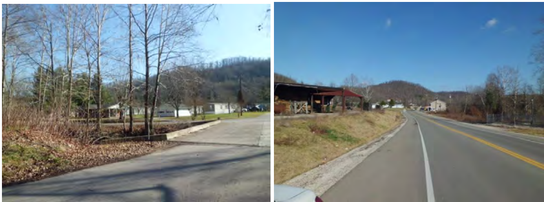
Figure 3.22. Photos from Dry Creek Watershed, DC-0.27.
