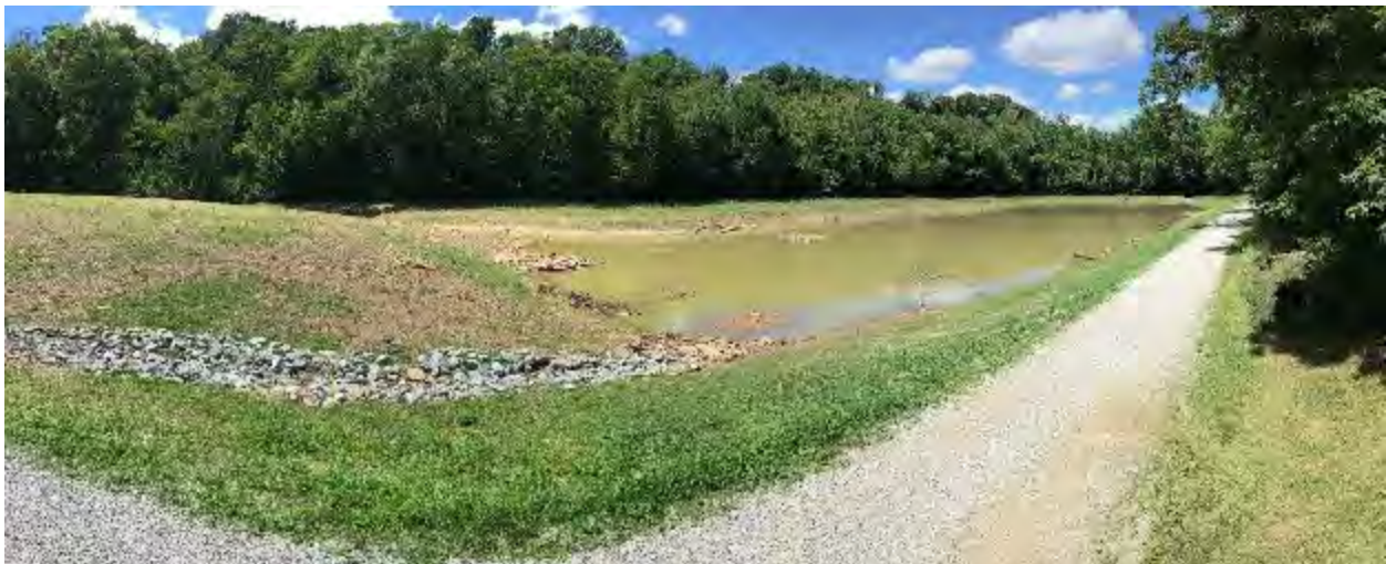
Bank full wetland recently completed at YMCA Camp Ernst on Gunpowder Creek
