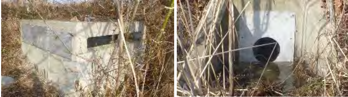
Example of storm water retrofits recently completed in Upper Woolper Creek
