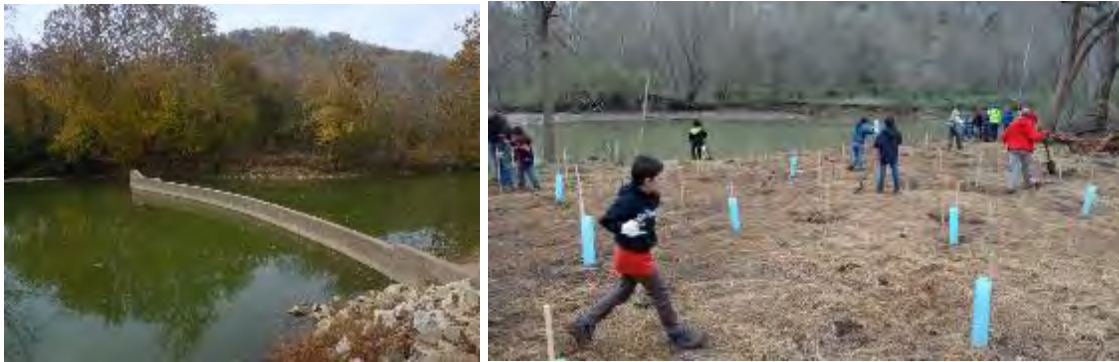
Low-head Dam removal at Camp Michaels on Gunpowder Creek
