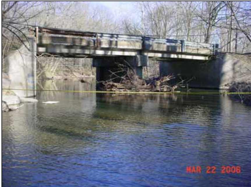
Oak Creek - This select site will catch the urban runoff (and outfall) from the majority of Junction City as well as an agricultural drainage. Located at 37.558674, -84.790585.
