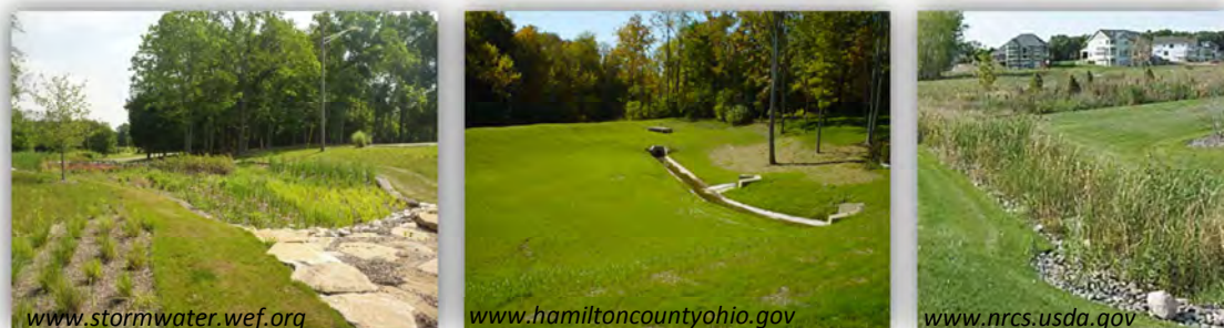
Figure 5-1: Stormwater BMPs: bioretention (left), detention basin (middle), and bioswale (right)
