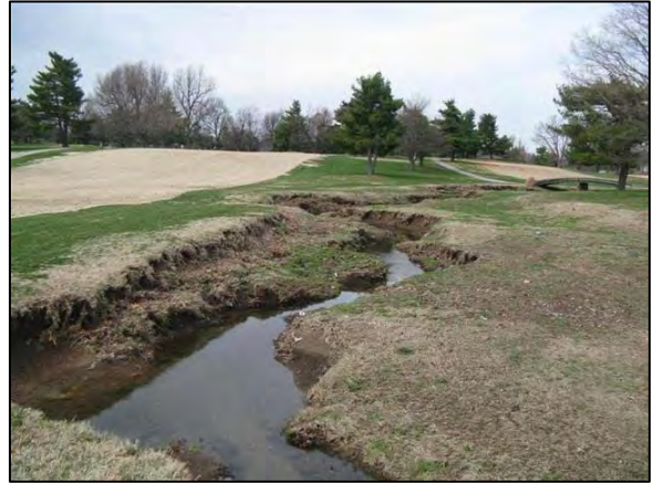
Erosion on Vaughn's Branch on Picadome Golf Course
