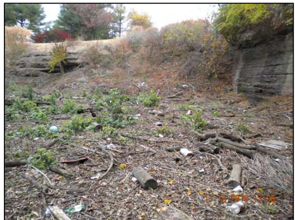
Debris Accumulation at Picadome Sinkhole Prior to Cleanup
