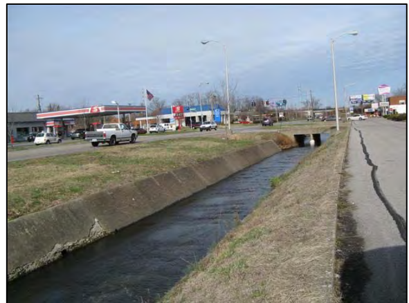
Wolf Run, Concrete Channel Beside Southland Drive
