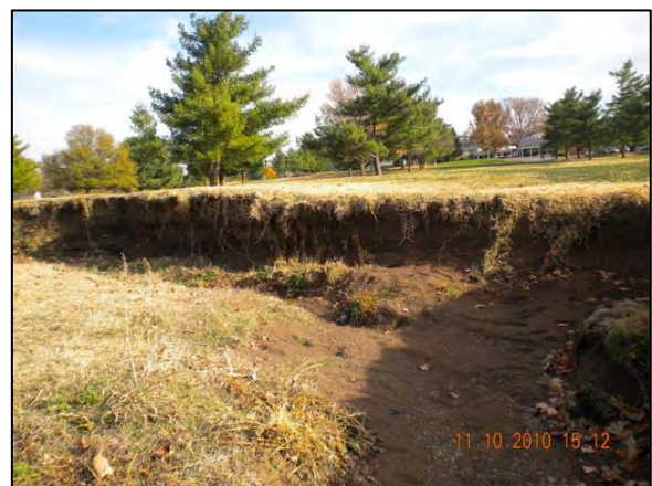
Severe Erosion on Big Elm Tributary near Picadome Sinkhole
