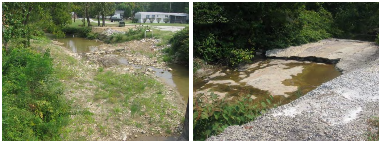
Figure 3.6. Examples of pipeline crossings on Dry Creek.
