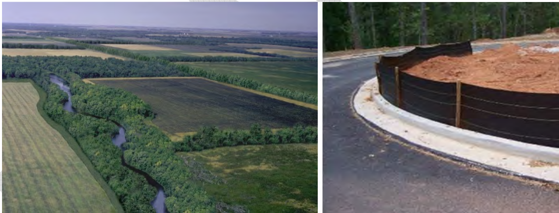
Figure 5.1: Riparian stream buffers and silt fences are structural BMPs that help protect water quality.
