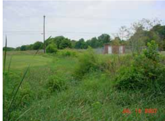
Pump station upstream of BB7
