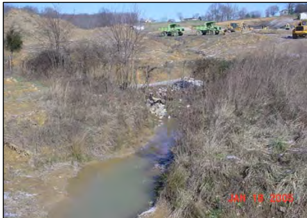
Construction Near Site 23A
