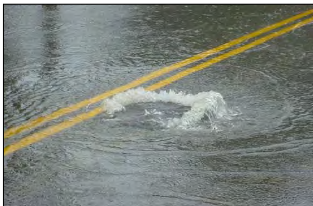
Sanitary Sewer Overflow
