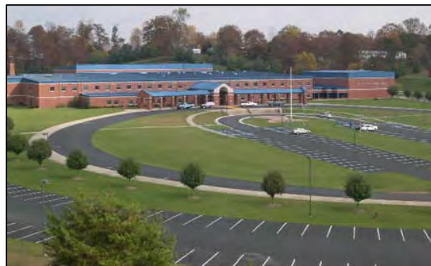
Impervious Parking Lot and Rooftop at North Laurel High School
