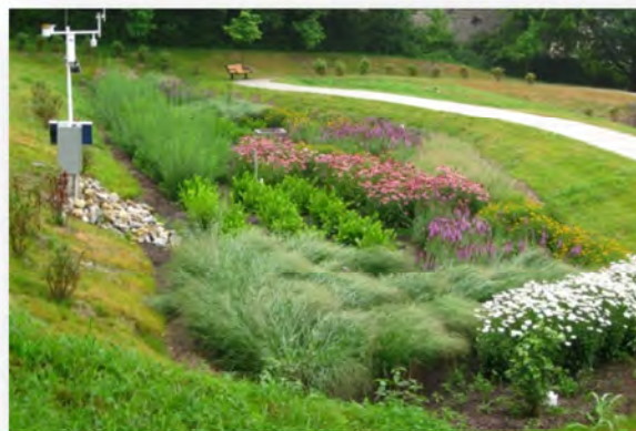
Figure 5-2: Bioinfiltration basin with native vegetation designed by Strand Associates to promote a more natural flow regime (Photo by Chris Rust)
