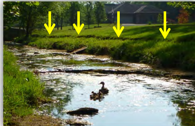
Figure 4-14: SFG 5.3-UNT 0.3 tension crack bank failure
