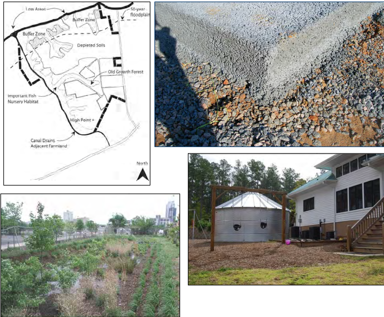
Figure 5-4. Examples of innovative stormwater design (clockwise from top left): Low Impact Development site planning, pervious pavement, parking lot draining to a bioretention cell, and cistern used for rain water harvesting (Source: NCSU (2009) and Heather Fisher, Tetra Tech)
