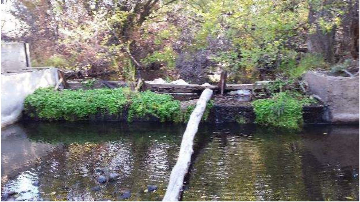
Photo 11 – Musgrave Diversion; Fish Ladder on Left (Aluminum Box)
