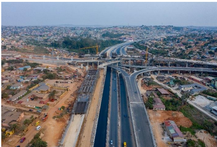
Pokuase Interchange (Accra Urban Transport Project)
