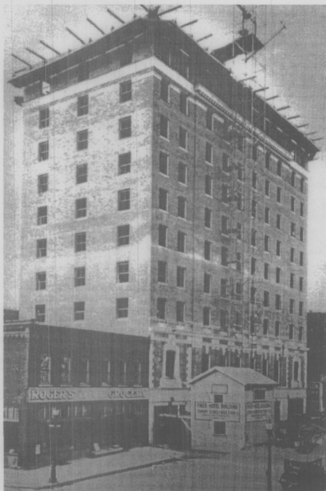
Figure Six. Construction of the Tiger Hotel, note the remodeled façade on the grocery store to the left.
